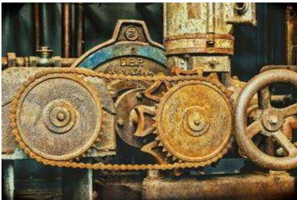
Figure 01 Corrosion general (rust) of a piece in steel
